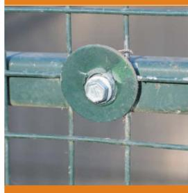
Figure 5: Fixing light mesh
