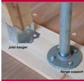
Figure 4A: Fixing method for timber Figure 4B: Fixing method for galvanised steel tubing
