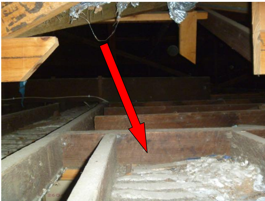
Figure 18: Uninsulated attic in Melbourne, Victoria.
