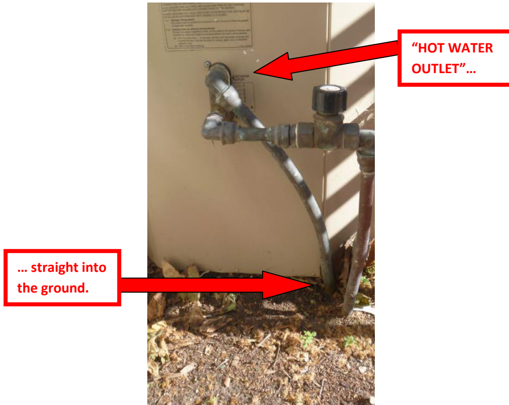
Figure 19: Uninsulated hot water outlet pipe running directly into the ground (Victoria).
